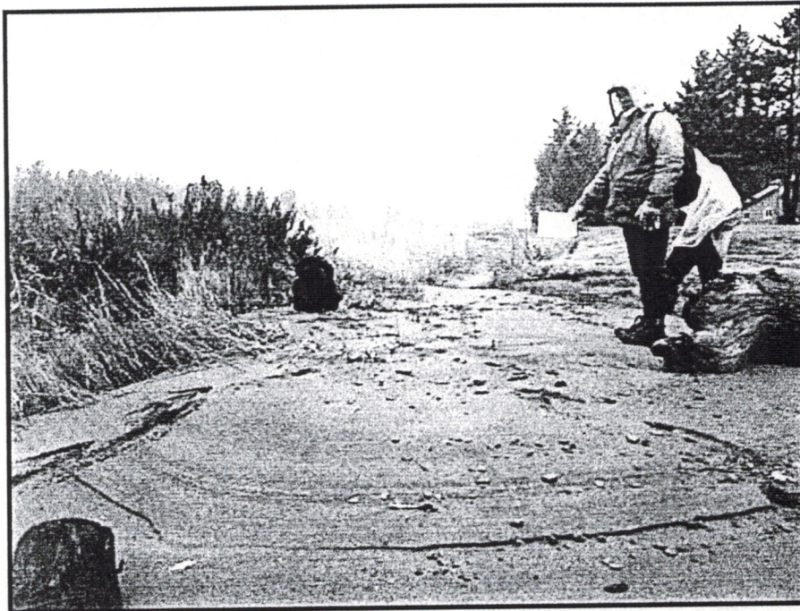
Figure 29. Serious sediment loading caused by a series of drainage ditches from a nearby farm at site 45.
