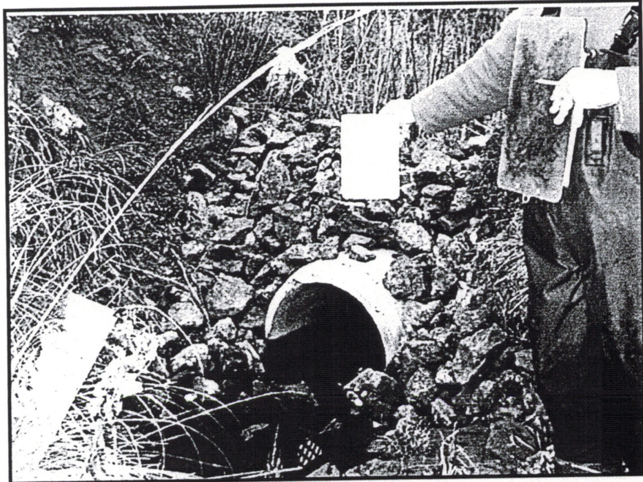
Figure 3. Cement culvert originating from Ditch Road at site 3.
