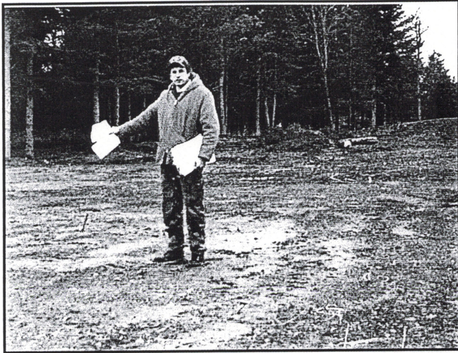
Figure 25. Small erosion ditches caused by bulldozing activities at site 39.
