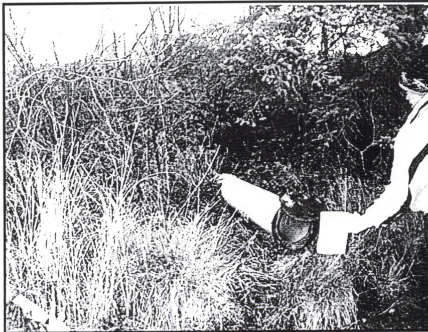
Figure 1. Plastic storm drainage pipe (with metal lid) originating from house at site 3.
