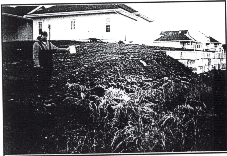
Figure 2. Concrete wall in front of house at site 2. There is approximately 30 meters of vegetation between the wall and the brook.
