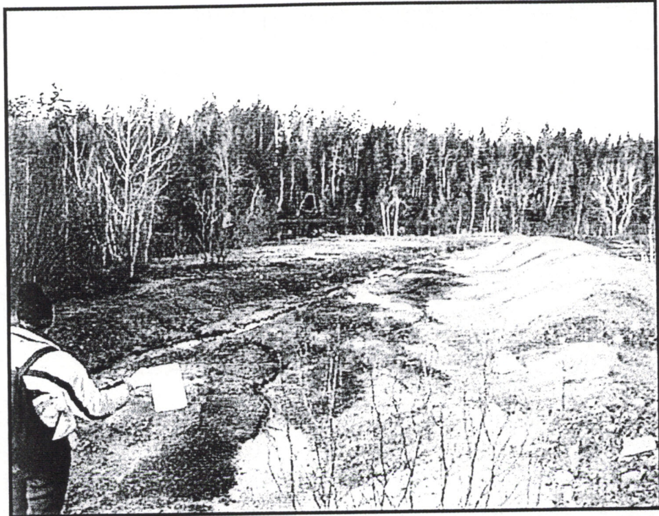
Figure 3. Small erosion ditch originating from abandoned pit at site 6.
