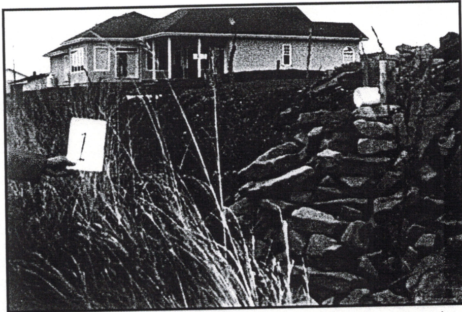
Figure 1. Two plastic drainage pipes originating from a house at site 1.
