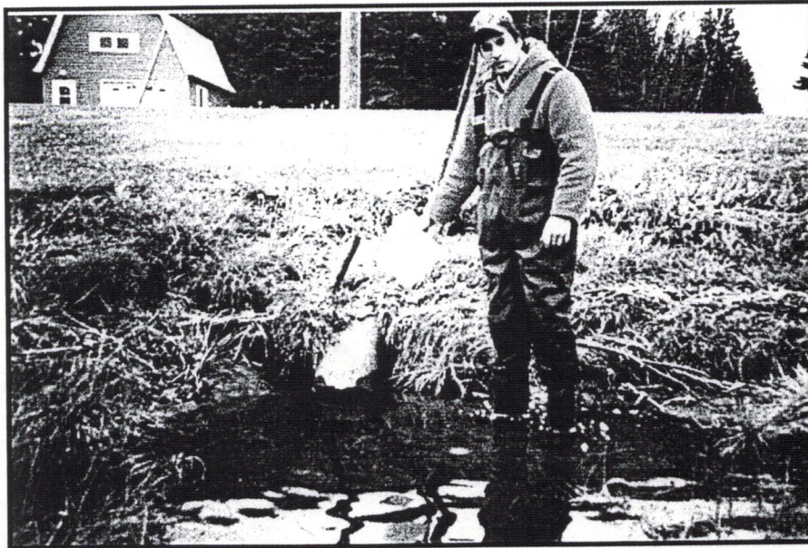
Figure 28. A cement culvert originating from a house's driveway ditch at site 44.
