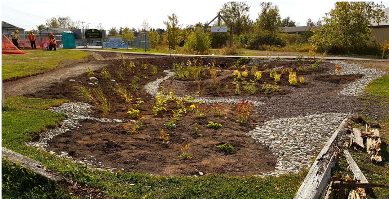
Figure 2: Rain garden construction photos, 2017
