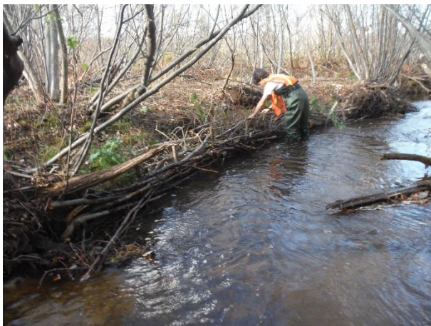
Figure 41: Building process of wattle fences, Cornwall Brook 2017
