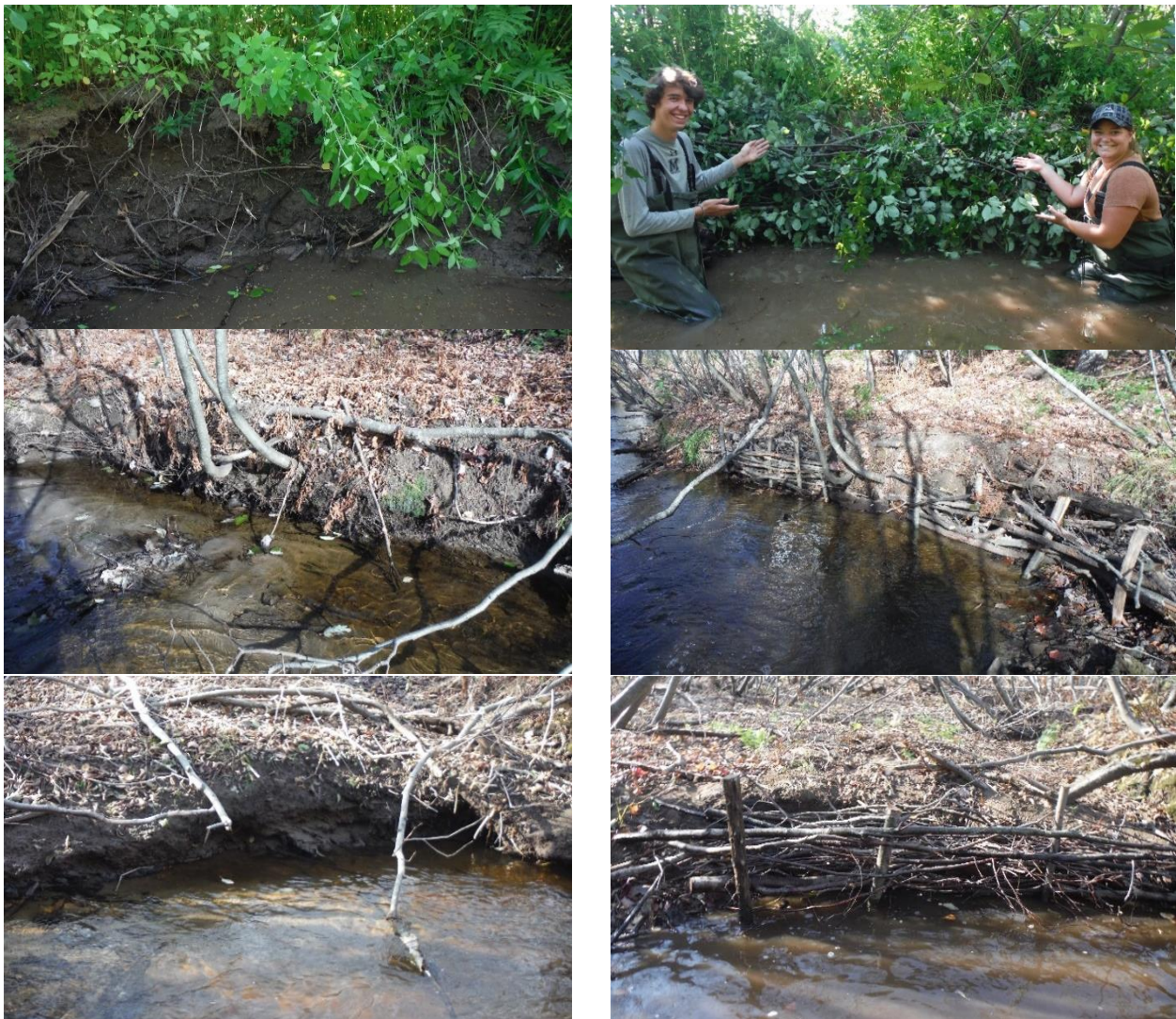
Figure 40: Before and after photos of the waddle fences, Cornwall Brook 2017
