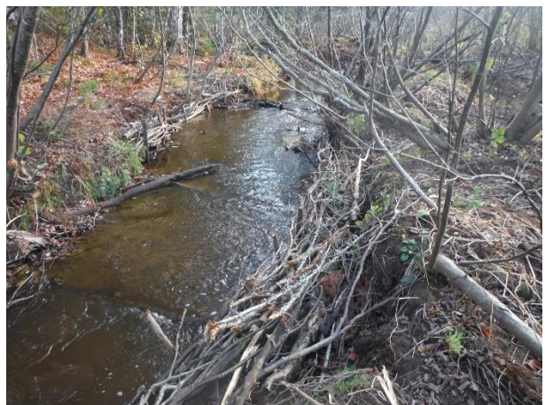
Figure 41: Building process of wattle fences, Cornwall Brook 2017
