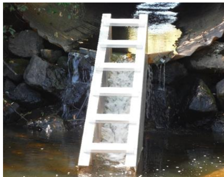
Figure 48: Fish ladder installed on the McQuade Brook.
